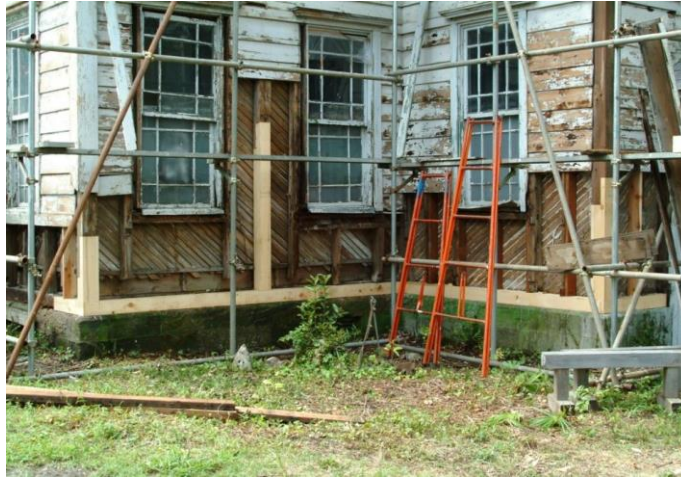
柱の腐朽 (→柱材のやり替え)
